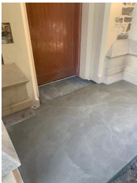
Completed NW step
